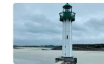
Restoration of the Lighthouse of Regeneron through FAREMER (RTE)
