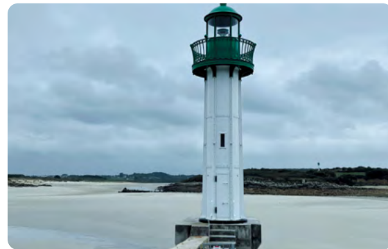
Restoration of the lighthouse of Mogueriec through FARÉMER, © RTE
